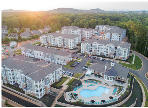
Beacon on 5th, Charlottesville, VA
