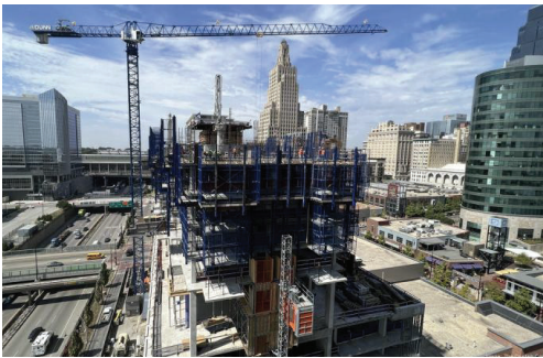
Three Light Tower - New construction Kansas City, Missouri
